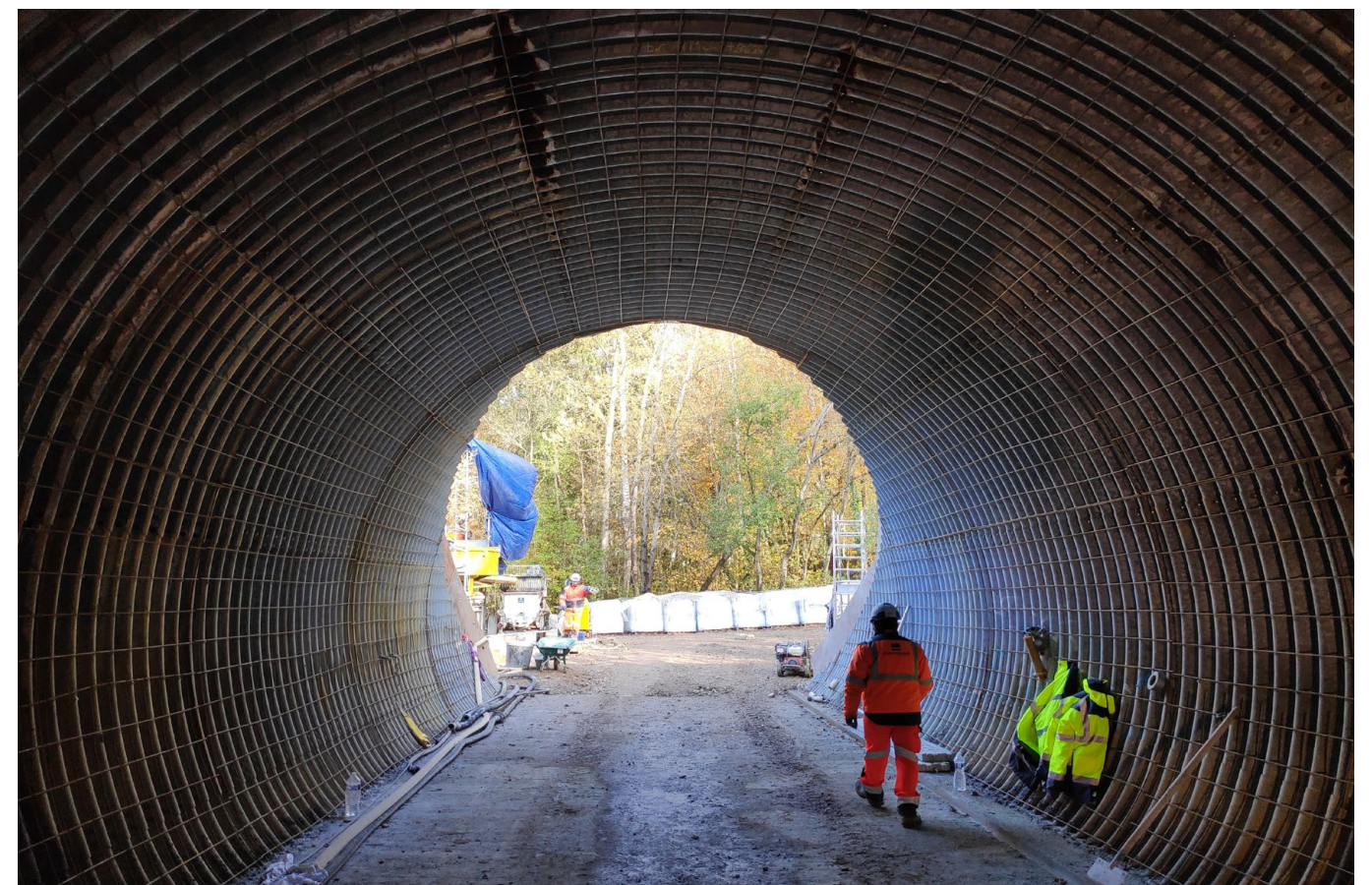
Sevenans metallic culvert, France, 2020 - Freyssinet
