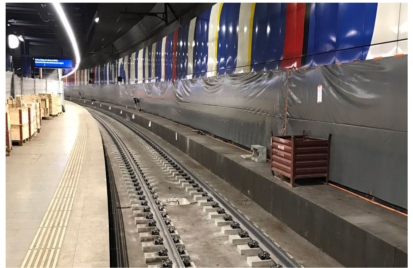
Zurich Airport railway station, Switzerland, 2019/2020 - ARGE FF Flughafen
