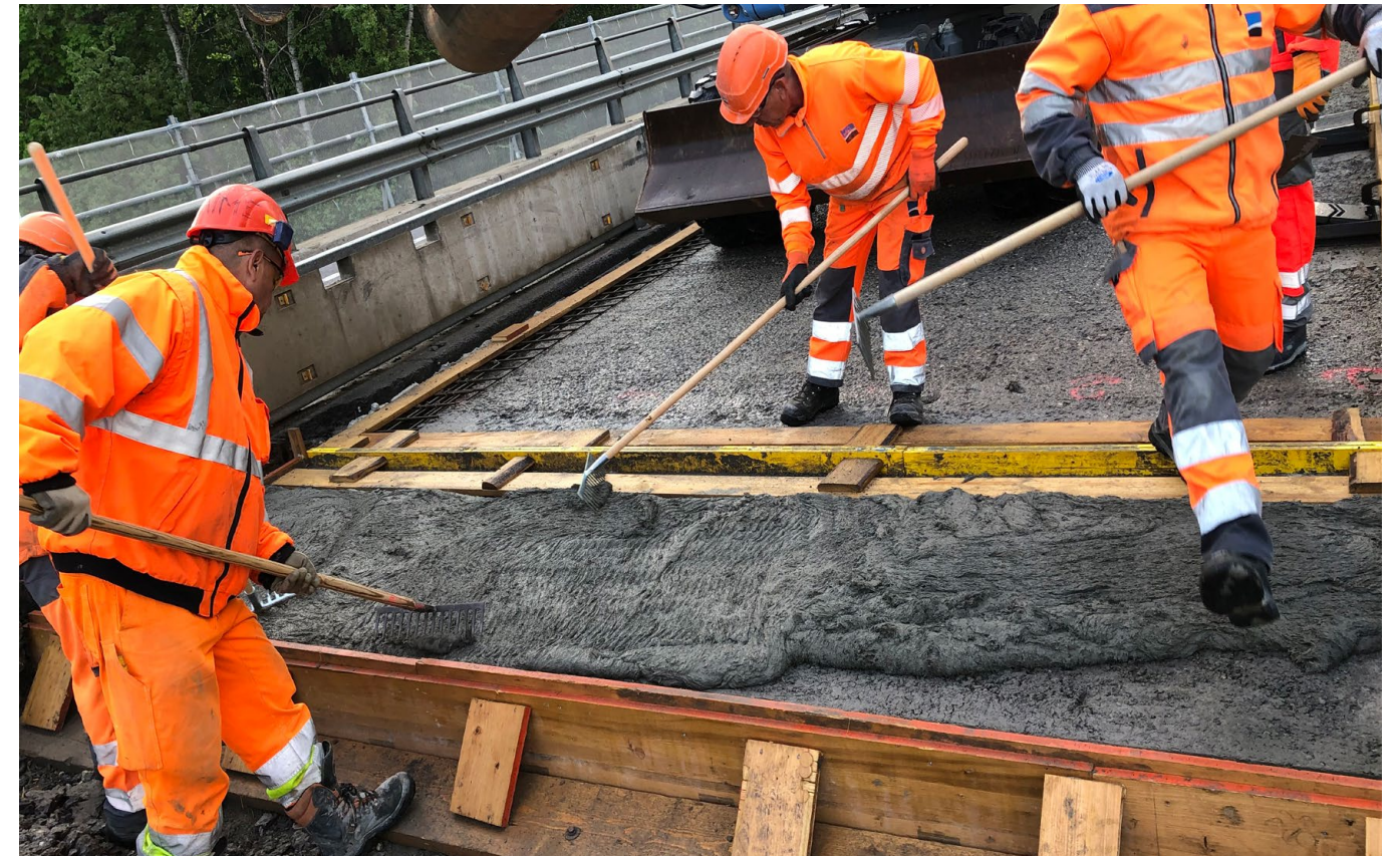
Des Fenils bridge, Switzerland, 2021 - Grisoni - Zaugg SA
