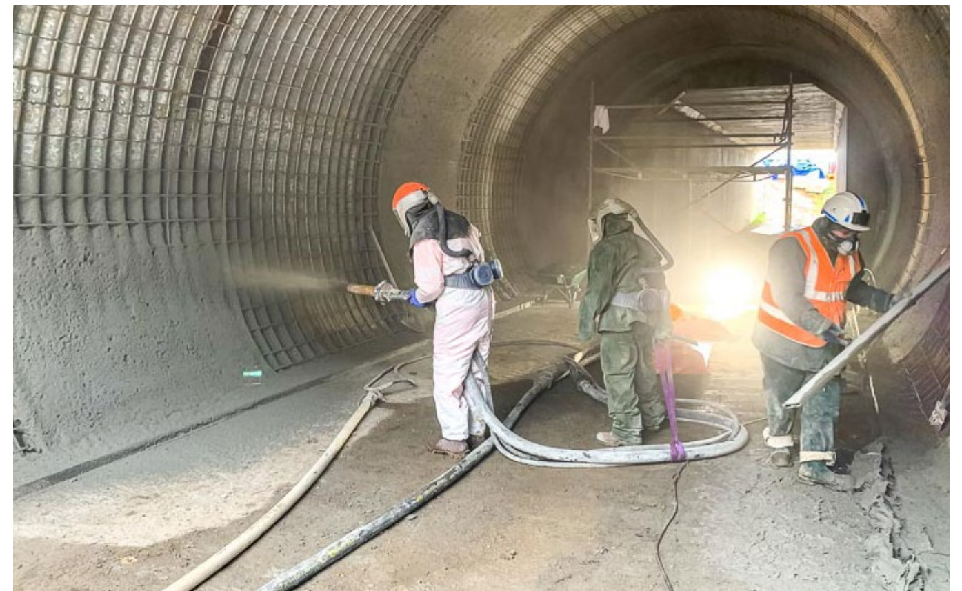
Barbazan metallic culvert, France - 2020, Freyssinet
