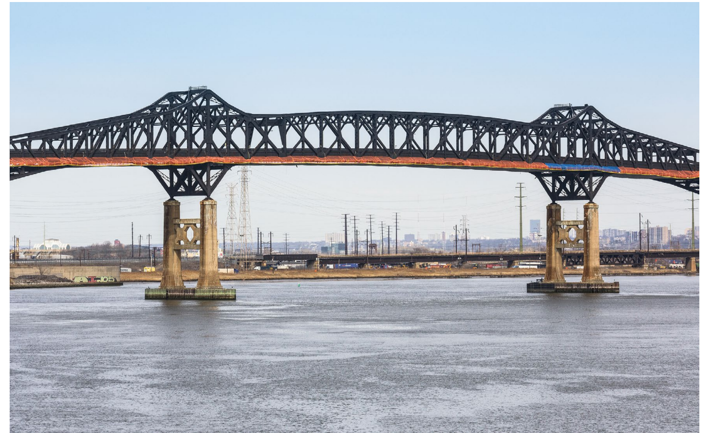
Pulaski Skyway, USA, 2018 - CCA Civil
