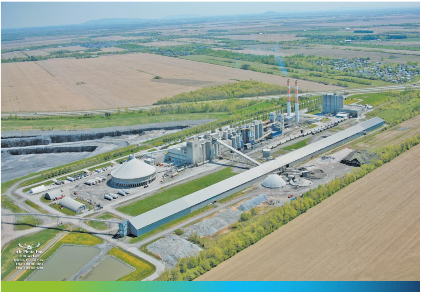
Lafarge St. Constant Cement Plant
