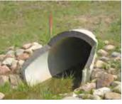
For larger sizes not listed above, box section beveled ends can be manufactured or pipe cut into 'Flare' as seen in the picture above. Please call for pricing.
