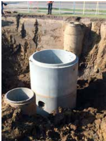
Jellyfish filter installation in St. Albert, AB. A JF8-6-2 was installed to obtain LEED credits and treat up to 32.5 L/s
