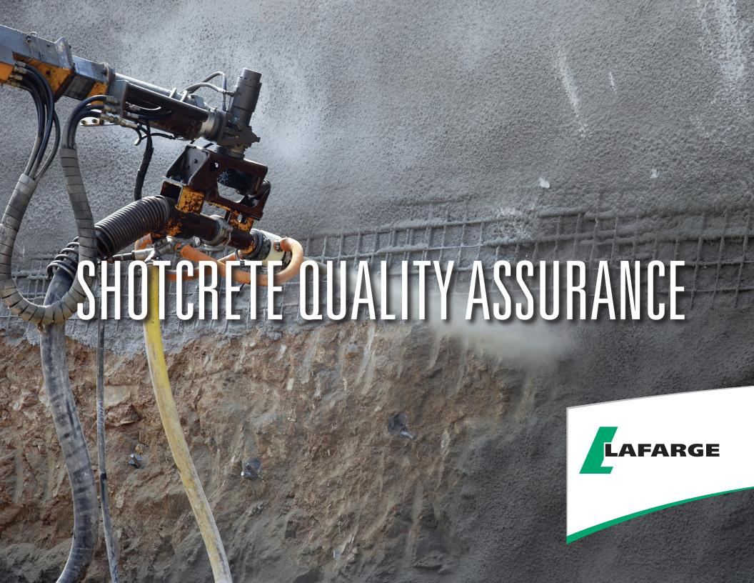
Lafarge has over 15 years experience partnering with mine owners to safely deliver high strength, wet Shotcrete mixes via slickline or borehole, without affecting performance and quality. Our wet Shotcrete for underground applications, which can include steel or synthetic fibers, has been tested and proven to provide adequate ground support to mines while keeping schedules tight. Compared to dry Shotcrete supply, Lafarge wet Shotcrete can significantly reduce costs and labour.
