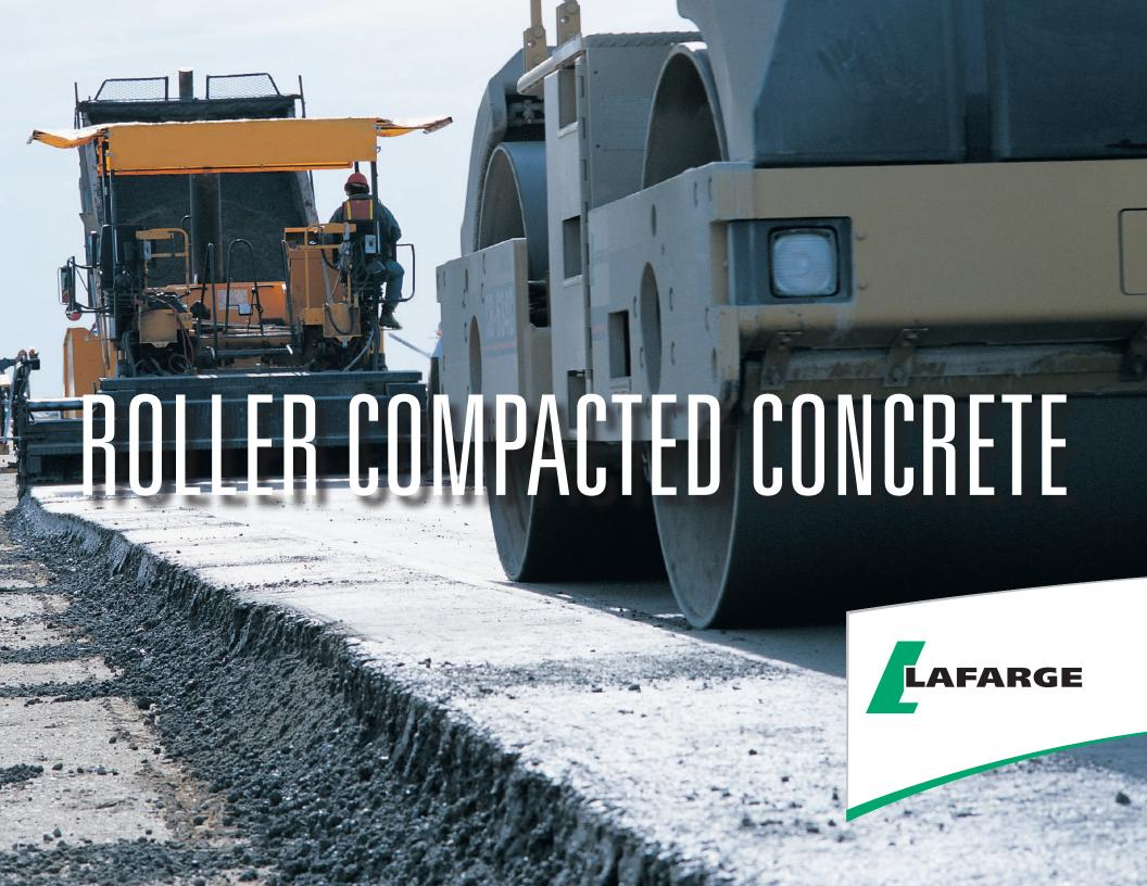
Roller Compacted Concrete (RCC) is a dry mix concrete which allows for placement without forms and is compacted by vibratory rollers. This provides a durable, low cost, high strength, industrial pavement with no steel reinforcement required.
