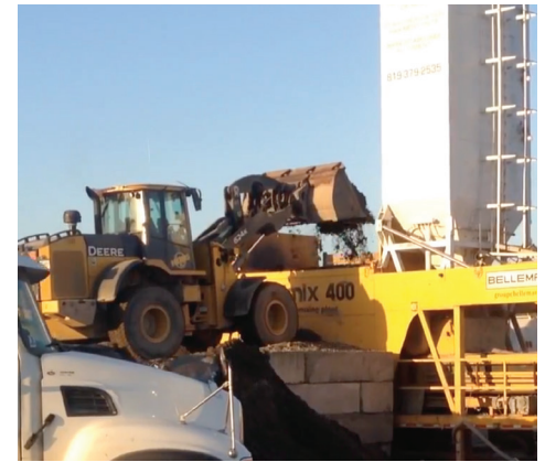
Contaminated material being placed into pug mill bin
