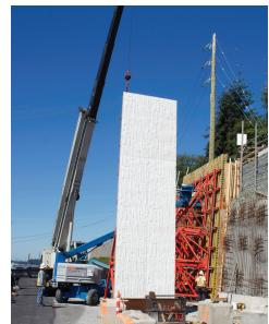
Road construction included, among others, associated concrete flat works, excavation, grading, asphalt and paving. Structural works consisted of constructing and assembling a single-sided gang-form mechanical formwork and applying decorative finish to concrete for the large grave-stake cast in place retaining walls. Construction of the Mechanically Stabilized Earth (MSE) walls, included both a precast panel wall and a green vegetative wall.
