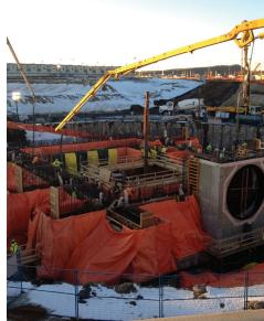
The next milestone was the pre-sink slip form in the South Shaft which took place in February 2013, followed by the North Shaft pre sink in June 2013. Both of these pours lasted approximately one week. Lafarge began supplying high early, high slump concrete for mine shaft liner in September 2013 and began providing 24/7 coverage to support the shaft sinking operations. The total shaft depths will be approximately 1036 meters. when completed at the end of 2017.
