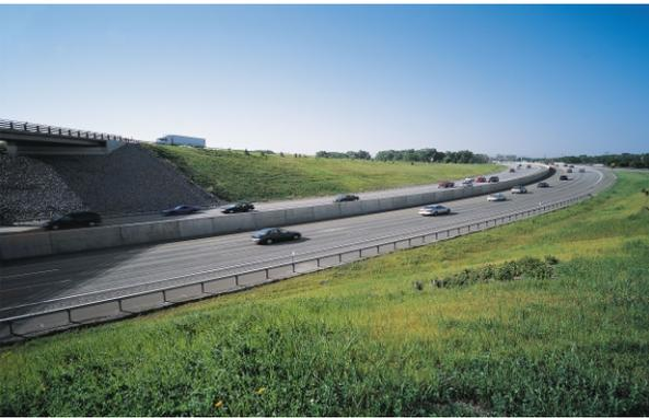
Durawhisper™ consists of a 10 mm, nominal size, dense graded asphalt mixture designed with 2 to 4% air voids. The aggregate particle shape and the design of the stone skeleton provide excellent rutting resistance, whilst providing excellent vehicle traffic noise reducing characteristics. Crumb rubber is added to the asphalt mix, which is beneficial for improved durability and long term performance, particularly when subject to heavy slow moving traffic.
