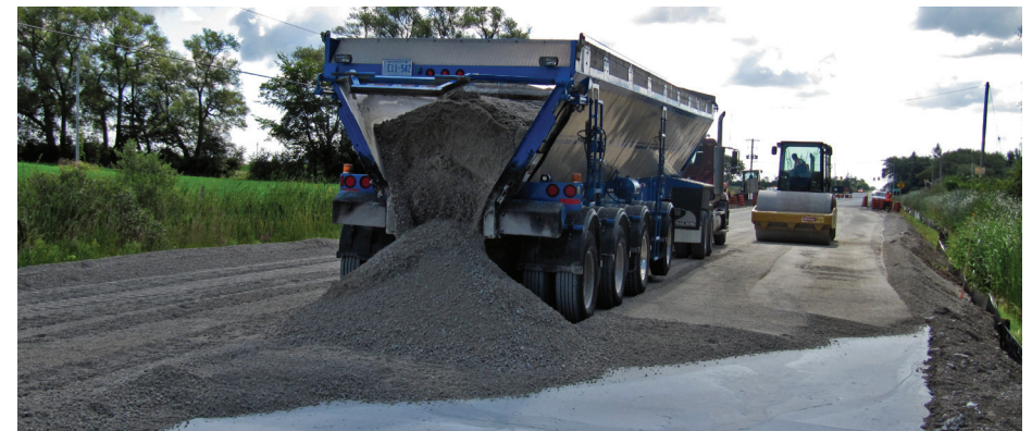
CEMATRIX™ used as lightweight fill for roadways
