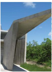
One of the most challenging aspects of the shower facility's design was this wall. Although, partially completed using the concrete from a previous supplier, it lacked the wood grain finish and knife's edge called for in the architect's design. By erecting the original forms over the existing wall and pouring a thin layer of Agilia® Architectural over top, Westland Construction Ltd. was able to complete the wall according to the architect's specifications.
