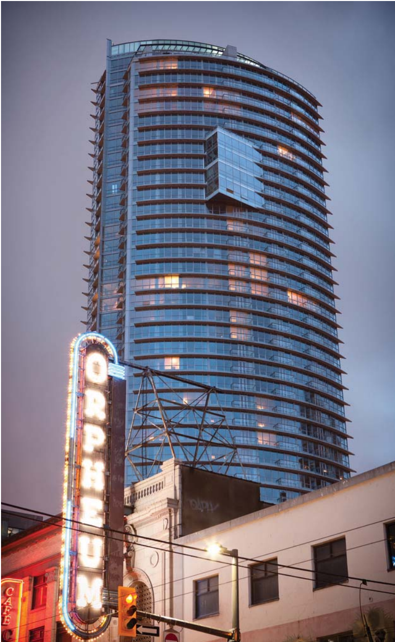
Capitol Residences, located next to the Orpheum Theatre in downtown Vancouver, is 42 storeys tall and contains 327 suites.
