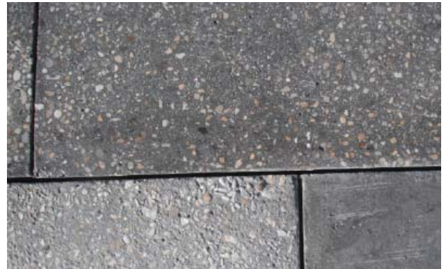
The East Village Riverwalk Phase I design incorporated 3 different Artevia® Colors: Executive Slate, Standard Slate, and Standard Limestone. It also called for 3 distinct stamps to be used on the panels along with exposed concrete and broom finishes. Two different kinds of aggregate, Edmonton Brownstone and Carseland, were used for the exposed concrete panels.
