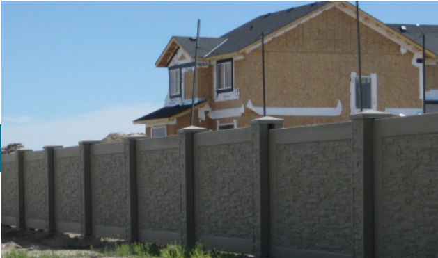
Using Chronolia® 4H helped Cast in Stone Fences by DDS Consulting accelerate their construction speed.
